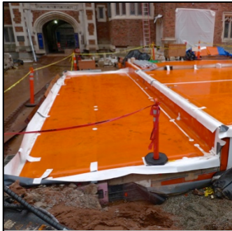
Waterproofing below Grade
