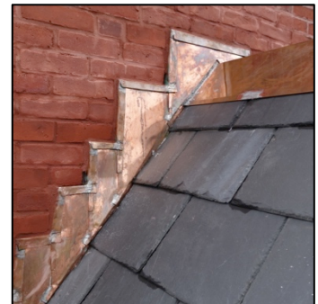
Slate and Metal Roofing
