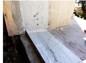
Fluid-applied flashings with an upstanding leg were installed under the new windows, to minimize water seeping directly under the sash.
