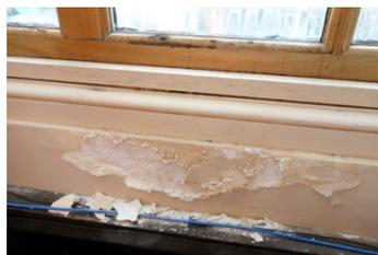
Leakage was causing damage to the plaster as well as rotting out the window sills.
