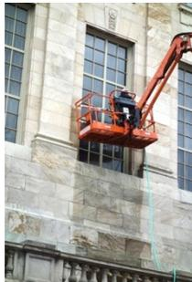
Water tests identified several different leakage paths, including glass perimeter leakage, leakage through mull posts and horizontals, and leakage at the sills and masonry, which had been dripping unseen into ductwork.
