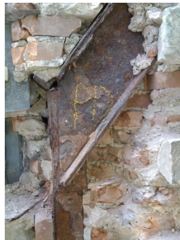
Electrochemical measurements were used to estimate how fast the rust was spreading. They showed little or no risk of corrosion on lower floors.
