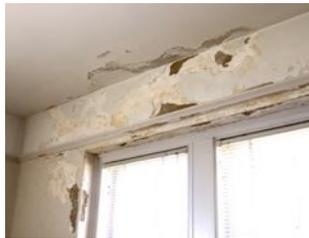
Leakage showed up in a variety of locations, for example, above window heads, and below window sills in projecting bay windows.
