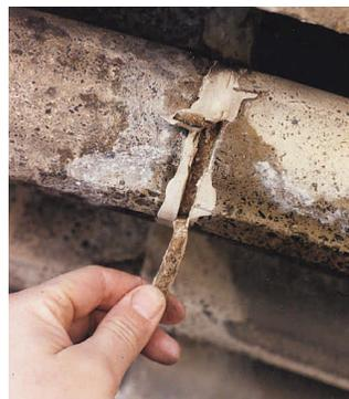
**Maintenance without Diagnosis** Makes a Problem Worse. A historic Gothic-style masonry building had been leaking for years. One of the symptoms was water and mineral deposits appearing around the mortar joints. In an effort to address the problem, the owners spent maintenance money to fill the mortar joints with sealant. The
