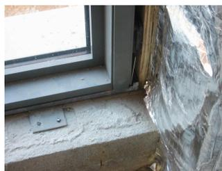
This photo shows a curtain wall sill corner in a building under construction, in which we can see sill fastener clips that penetrate the sill flashing, backer rod braided like a rope, and flashing corner
